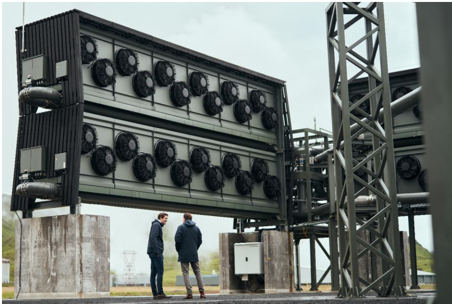
Climeworks' direct air capture & storage plant Orca permanently removes CO 2 from the air, © Climeworks.
